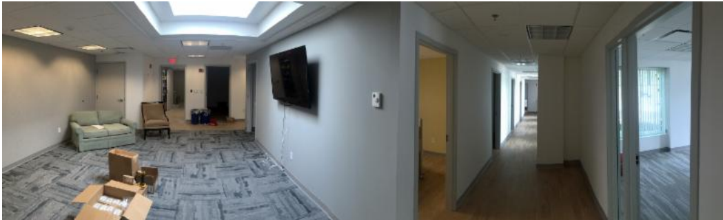
The new Health and Wellness Center nears completion.
